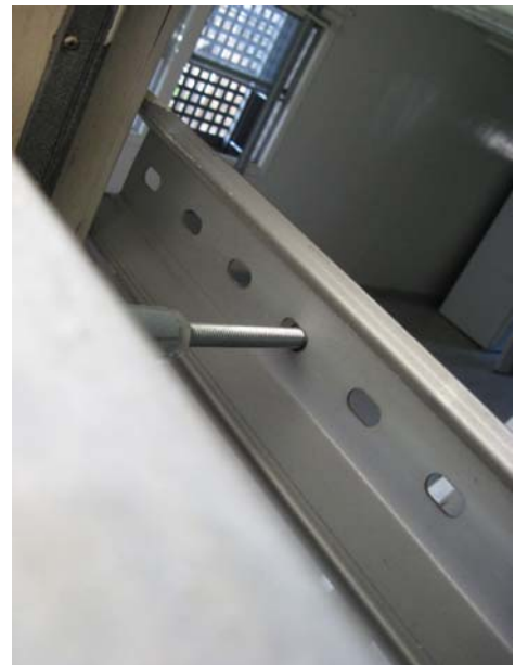
Door Attachment from inside
