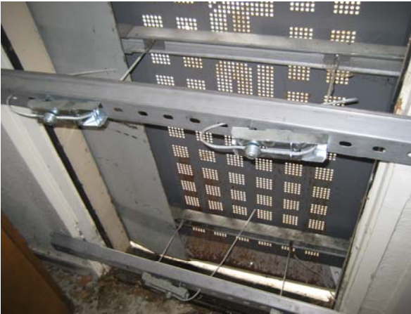
Cable Adjustment Bracket
