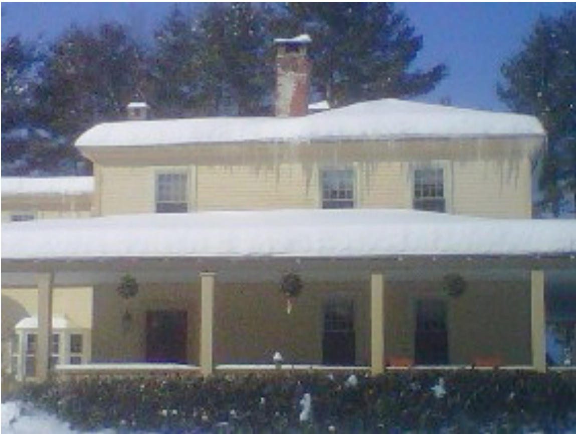
This photo displays both a Warm Roof (on top) and Cold Roof (porch)
