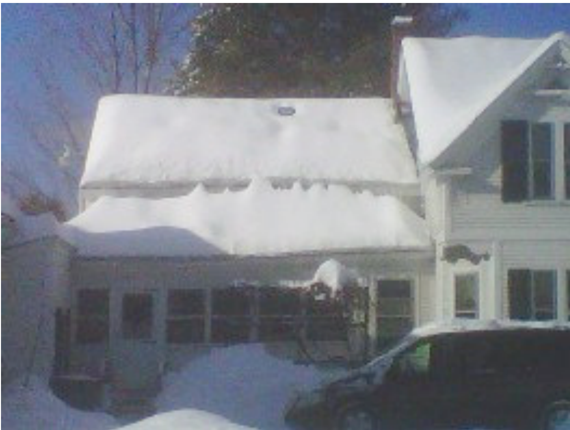
In this photo: Older Farmhouse with a noted sagging porch roof
