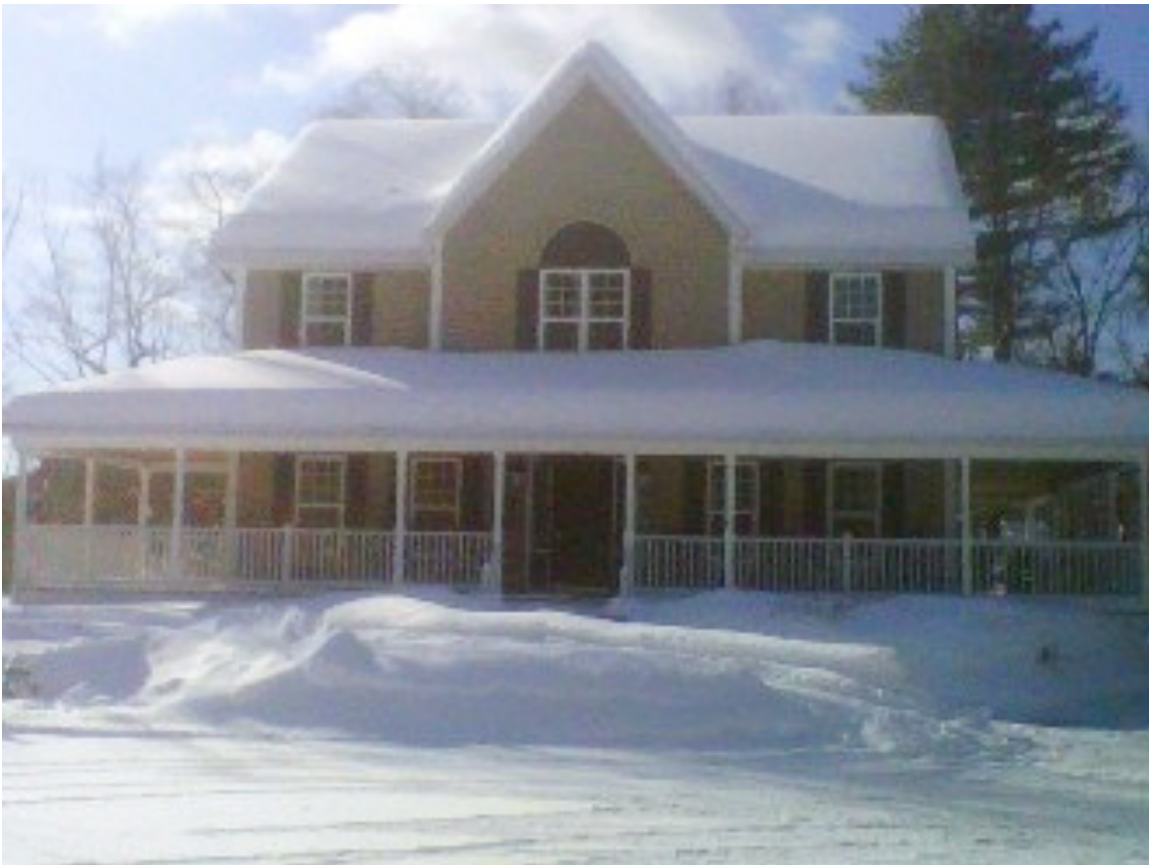
Lightweight Construction – Very Large Farmers Porches are great snow load collectors
