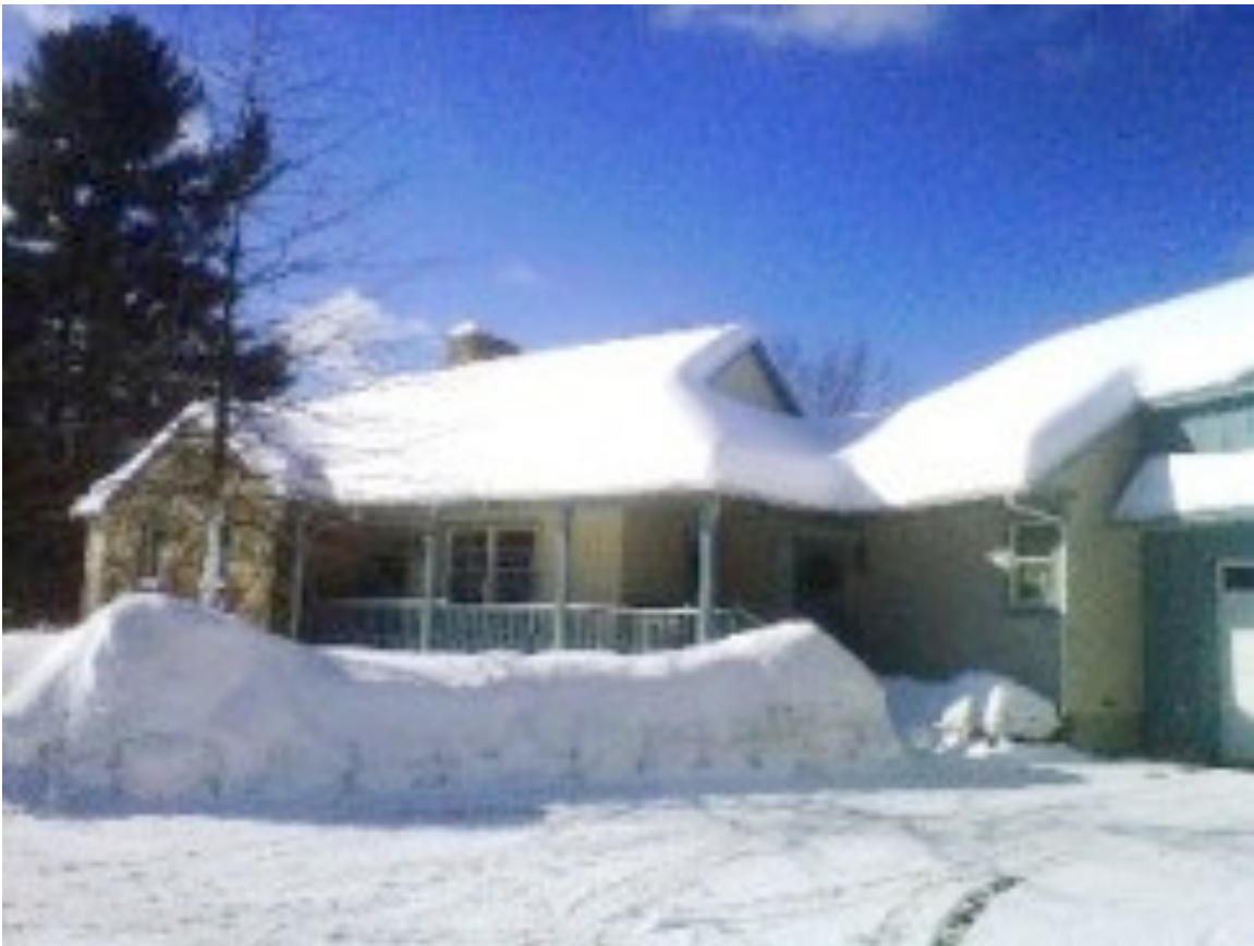
Farmers porch buildup that hinders normal 8/12 pitch roof snow slide
