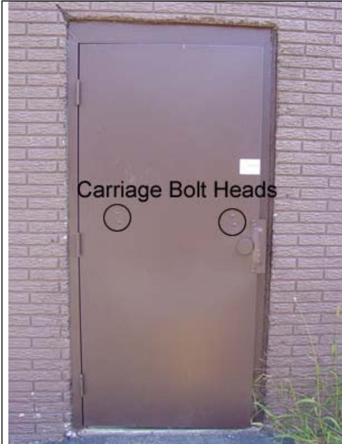
Exterior view with door closed. Note 4 visible carriage bolt heads, indicating the possible presence of a door bar. Also note the lack of exterior doorknob and added strike plate protection.
