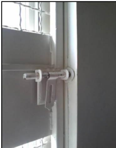
Picture 5. The locking mechanism. When secured, there will be a pad-lock attached.
