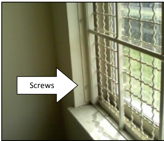
Picture 3. This side of the window gate does not open. See screws holding frame to wall.
